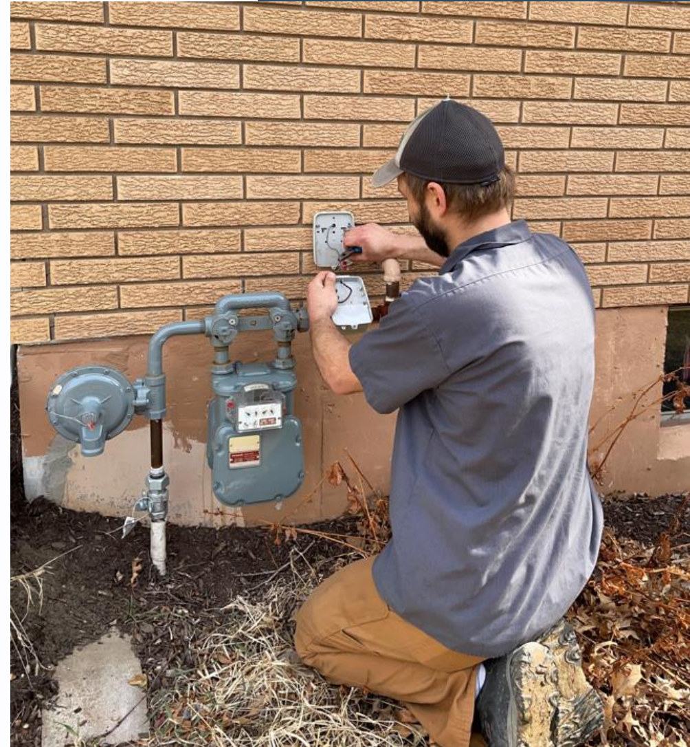
Danny Petersen installing new MIU
