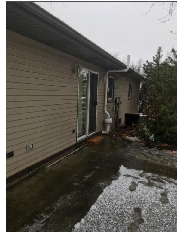
Radon Mitigation System
