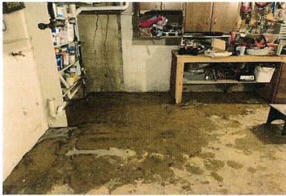
Water returning to basement through sewer line
