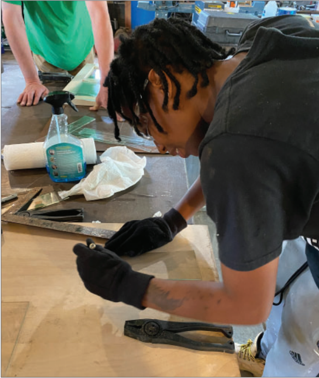
Mikaila cutting glass during window restoration training at Four Mounds.
