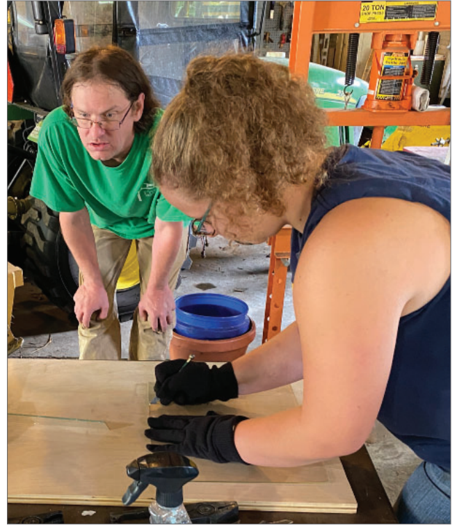
Liz cutting glass during window restoration training at Four Mounds.
